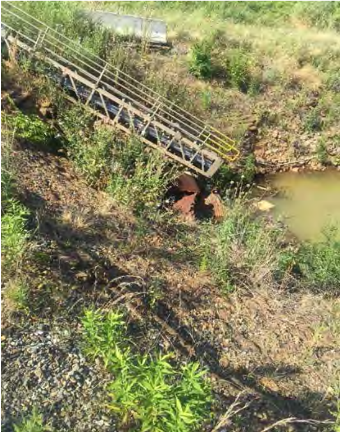
Photograph 9 – View of pipe that carries flow from an offsite location into the channel.
